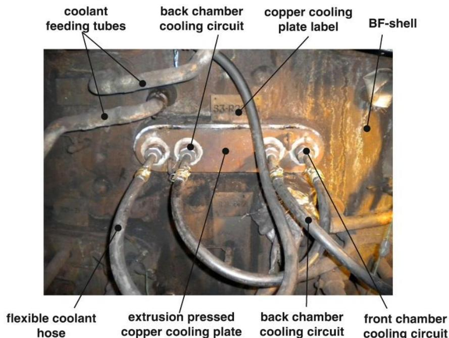
*Fig. :5 New-Copper Plate Cooler installation in the Cooling Row 22 of Blast Furnace A Lower Stack*
