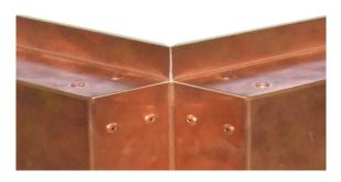
Examples for the rivet arrangement as a function of the corner cut for peripheral bent edge formats
